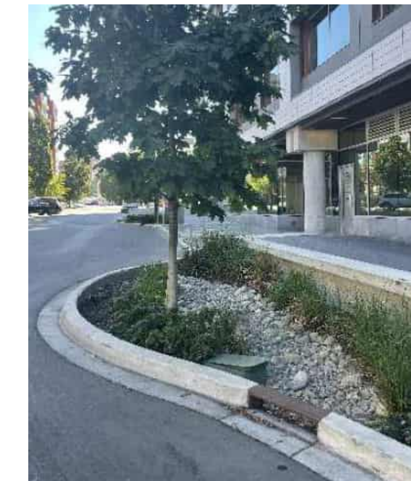
2. Street surface runoff collection into rain garden.
